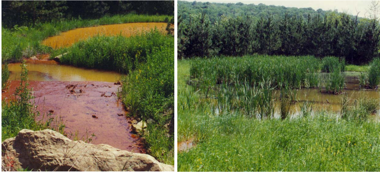
Figure 3: The Ellick I passive treatment system
