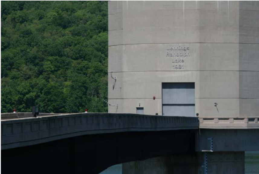
Figure 9: Bridge to intake control tower at Jennings Randolph Lake
